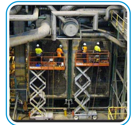
Condenser tube repair/replacement heat transfer margin recovery project.
